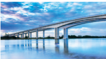
Monitor infrastructural deterioration in bridges
